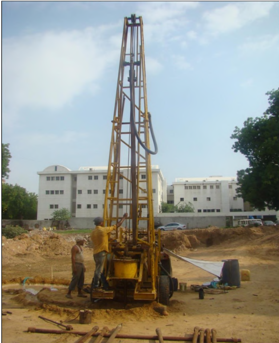
Fig. 6.3.13: Field Photograph of Mud Rotary Drilling Machine at V. S. Hospital site, Paldi
